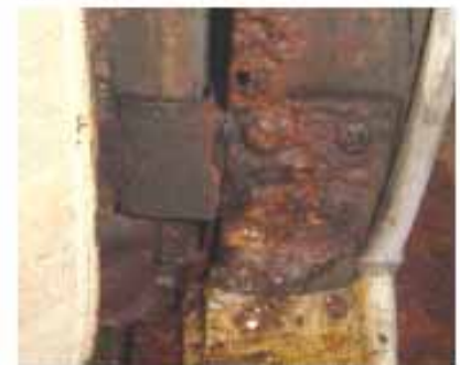
The rusty door hinge (photo courtesy John Egger)
